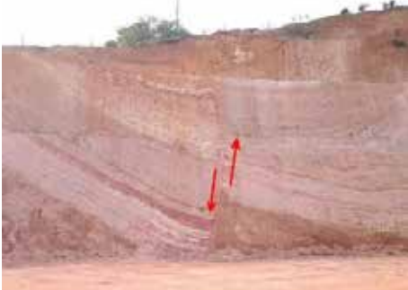
Figure 4: Sectional view of a fault exposed in a cut slope face closer to the Durekkanda
