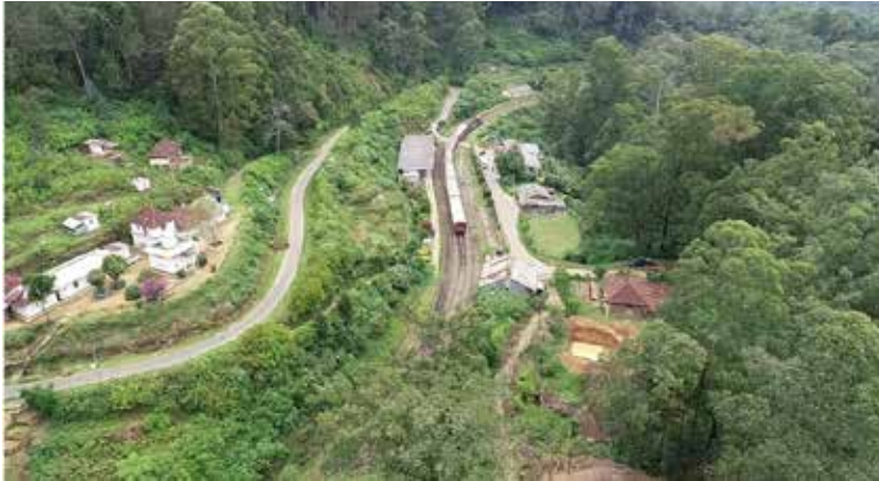
Figure 1: Ohiya Railway Station & Surrounding Area
