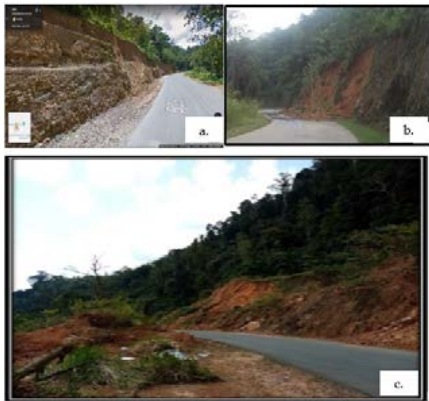
Figure 2: Initial rock cut slope failure in 2015 (a) Progressed cut slope failure in 2016 (b) cut slope failure developed into a landslide in 2017 (c) in Durekkanda
