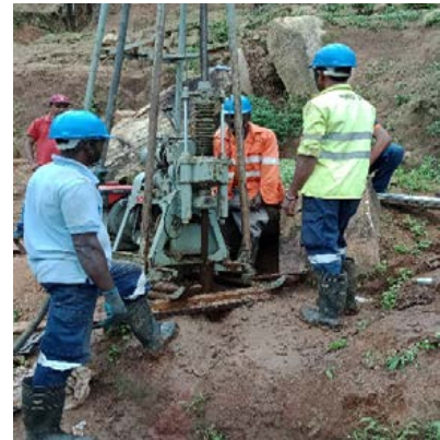
Figure 3: Installation of Inclinometer
