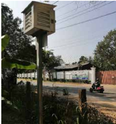
Figure 04: Installation of Monitoring Unit at Anuradhapura Urban Area
