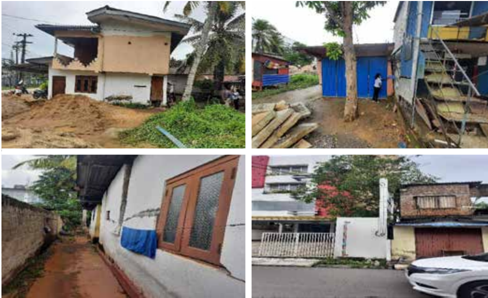
Figure 01: Adjacent building failures and settlement cases around Galle Municipal area
