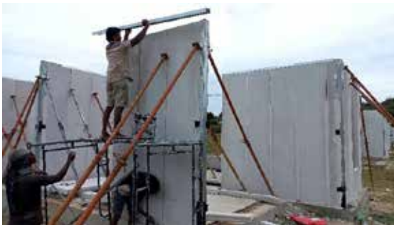
Figure 06: Connection between panels
