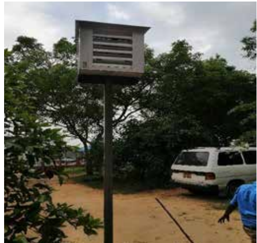
Figure 03: Installation of Monitoring Unit at Kurunegala Urban Area
