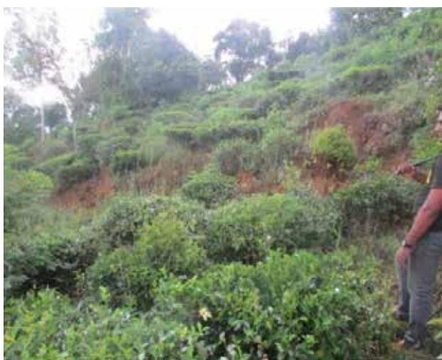
Figure 01: Landslide occurred in a Tea land (Pinnawala).
