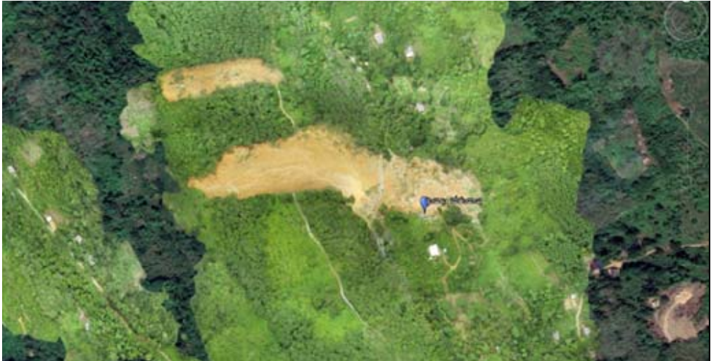
Figure 03: Drone image of the landslides
