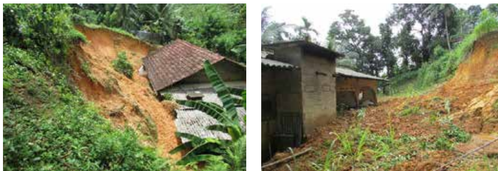
Figure 02: Several cutting failures and destruction caused in Nagoda DSD
