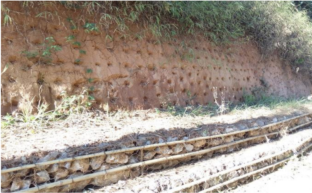
Slope face is drilled for growing plants. The toe of slope is strengthened with a gabion wall
