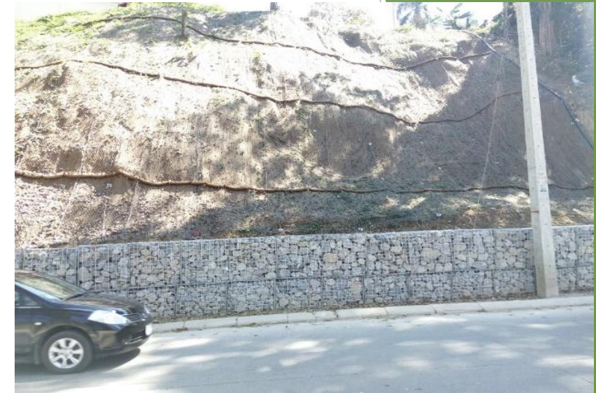
Gabion wall acting as a toe support
