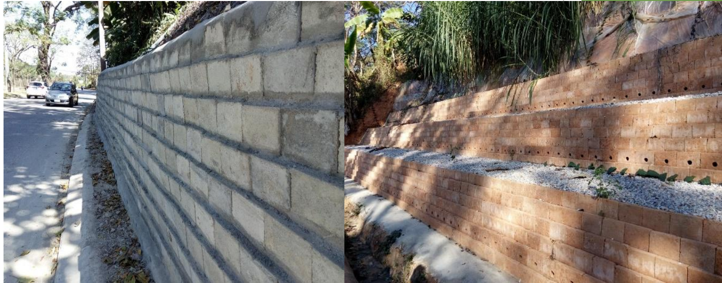
Walls constructed using TOR blocks
