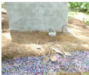
Figure 6: Wall with rubber trench
